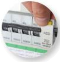
Consumer unit (fuse box or trip switch)-
